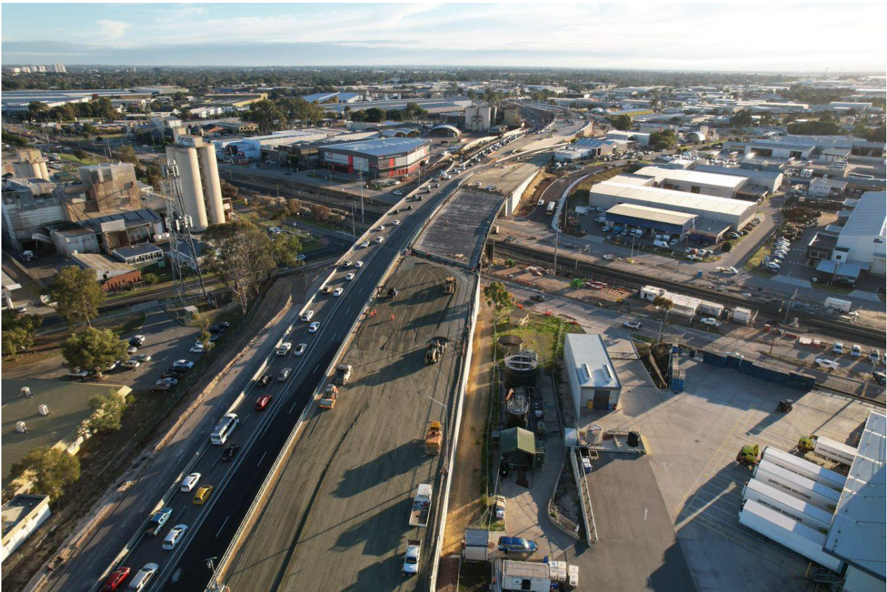
Figure 6 Industrial Area Adjacent to the Project, photograph of Bridge 1882 over rail facing north.
