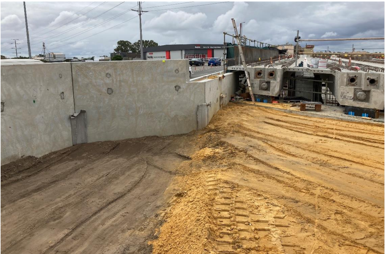
Figure 11 Retaining wall backfill with recycled sand
